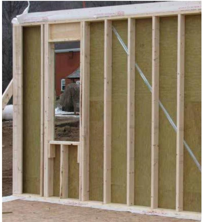
As an exterior insulation, ROXUL COMFORTBOARD 80 is fastened to the exterior OSB/plywood sheathing or structural stud wall and is designed to provide increased thermal performance to the building envelope
