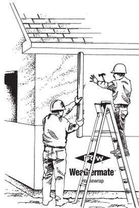
3. With roll straight and plumb, attach trailing end of Weathermate™ Brand Housewrap to framing members or nail-base sheathing. Unroll around corner, keeping membrane level, tight and flat. Wrap completely around building, covering windows and doors. Tuck tightly into inside corners using flat edge of 1x4 or similar.
